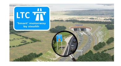
"In common with most A-roads, the A122 would operate with no hard shoulder but would feature a 1m hard strip on either side of the carriageway. It would also feature technology including stopped vehicle and incident detection, lane control, variable speed limits and electronic signage and signalling" - Paragraph 2.2.6 of Section 6.2 of the Transport Forecasting Package.
